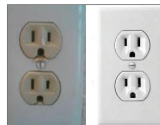
*The left outlet, or receptacle, has been damaged, while the right receptacle remains intact.*
