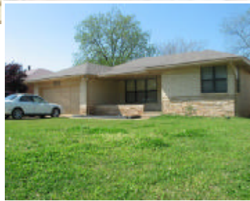
Pictured Above: LaShawn Williams stands at the front door of her new home (inset).
